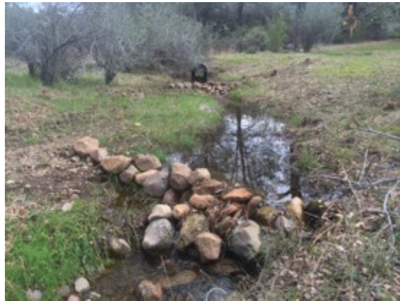
Picture 16: Resident lines a creek bed with boulders Picture 17: Check dams built by residents
